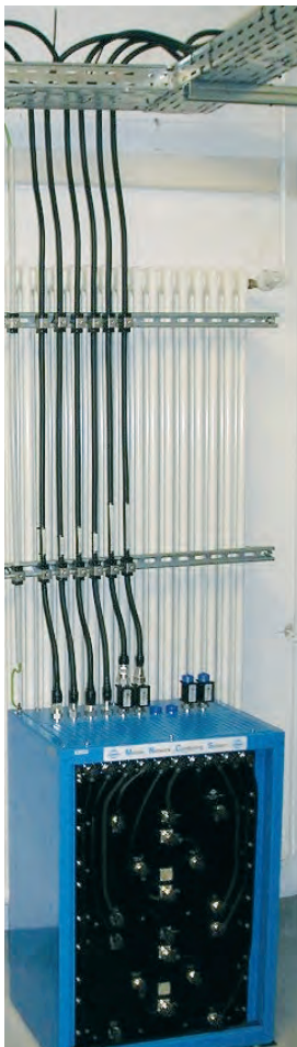
MNCS®-Schrank im Innenbereich MNCS® rack as compact wall-mounted solution
